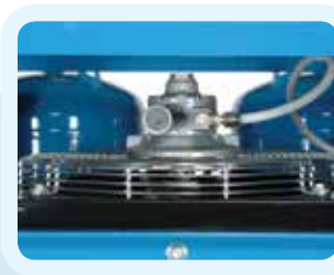
Air Powered After-Cooler
